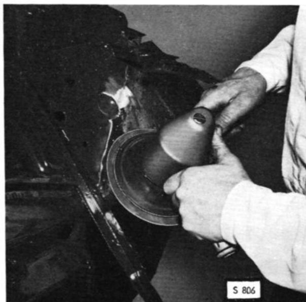
GRINDING AWAY WELD REMAINS
