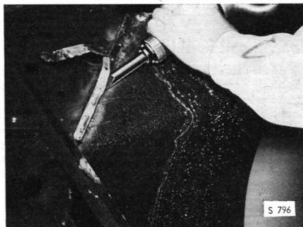
CHISELING OFF REMAINING METAL STRIPS
